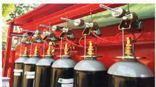
High Pressure CO 2 Fire Fighting System
